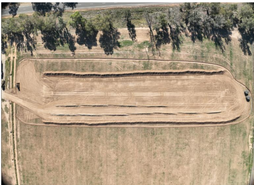
Top view of the earthworks at the NERPS
