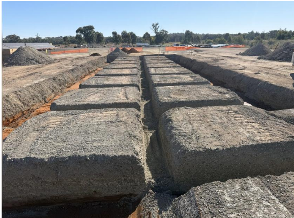
Footing for the slab at the ARPS
