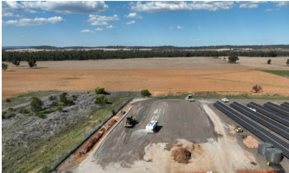
Earthworks at the ARPS
