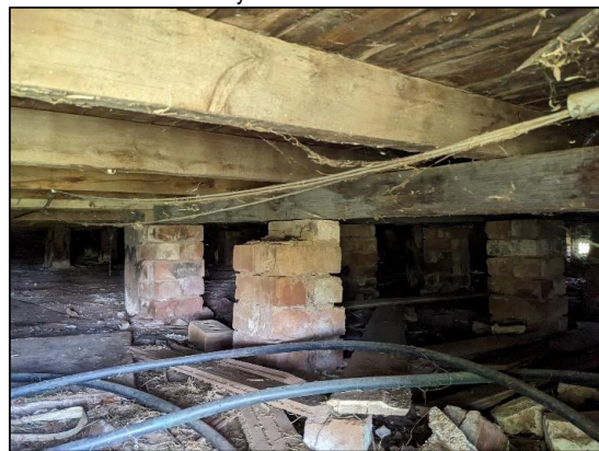
Footings presenting signs of mechanical breakdown
