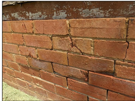
Brickwork presenting white staining and signs of mechanical breakdown due to salt crystals
