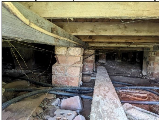
Footings presenting signs of mechanical breakdown
