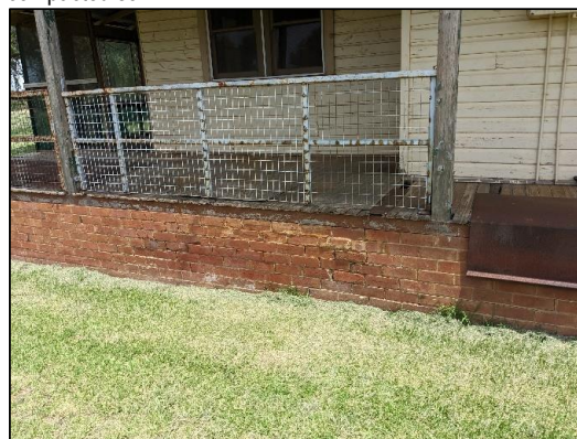
Base of dwelling presenting dampness "tide marks" and signs of mechanical breakdown due to salt crystals
