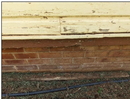
White staining due to salt crystals at the base of the dwelling
